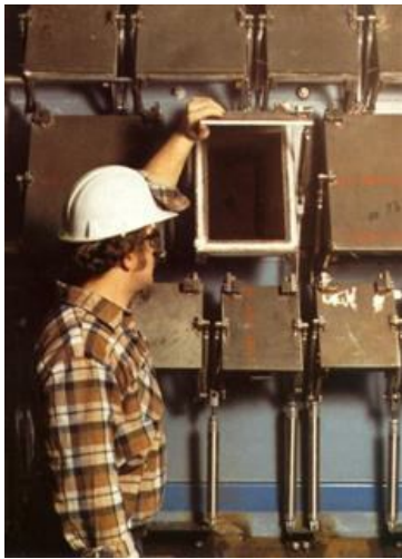
230 ® retorts operate at 2100°F (1150°C) with a hydrogen atmosphere (inside) and combustion products outside.
